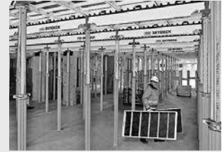
Slab Formwork
