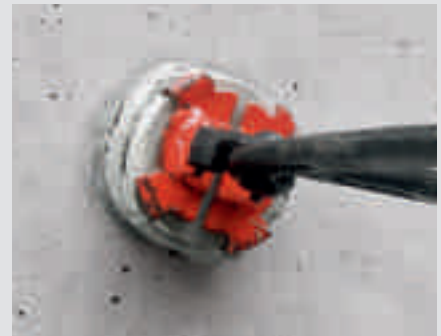
Insert the concrete cone into the pocket, and turn slightly several times to ensure that the sealing compound is evenly spread.
