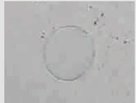
A clean and tight tie point with the PERI Tie System.
