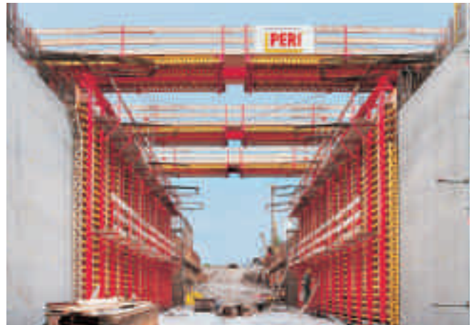
B311 Local Bypass Tunnel, Ertingen, Germany.
