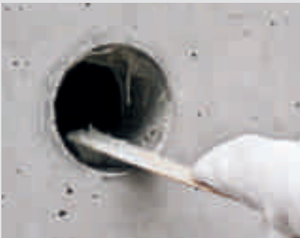
Coat the cleaned pocket sparingly with the sealing compound.
